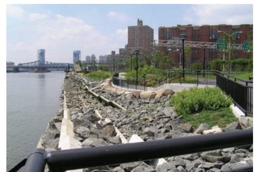
Harlem R. Park looking north from 140th St. after construction by EDC, 2009
